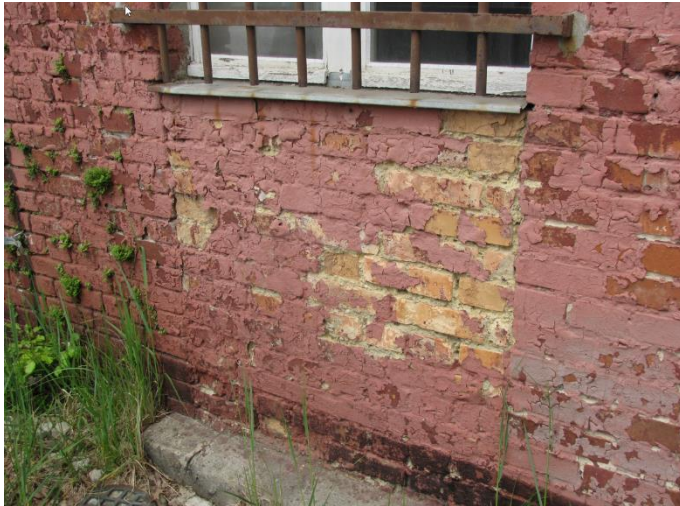
Fig. 3 Example of dense coatings to be removed
