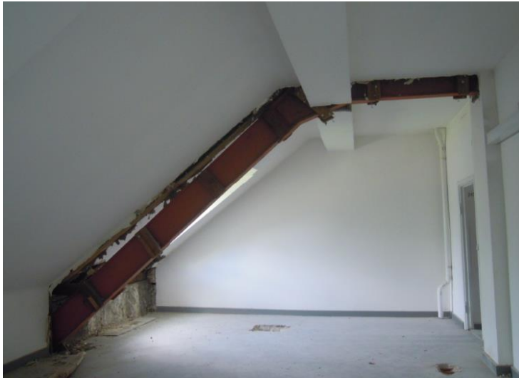
Fig. 21 Steel frame construction in the thermal plane with integration into the reinforced concrete jamb
