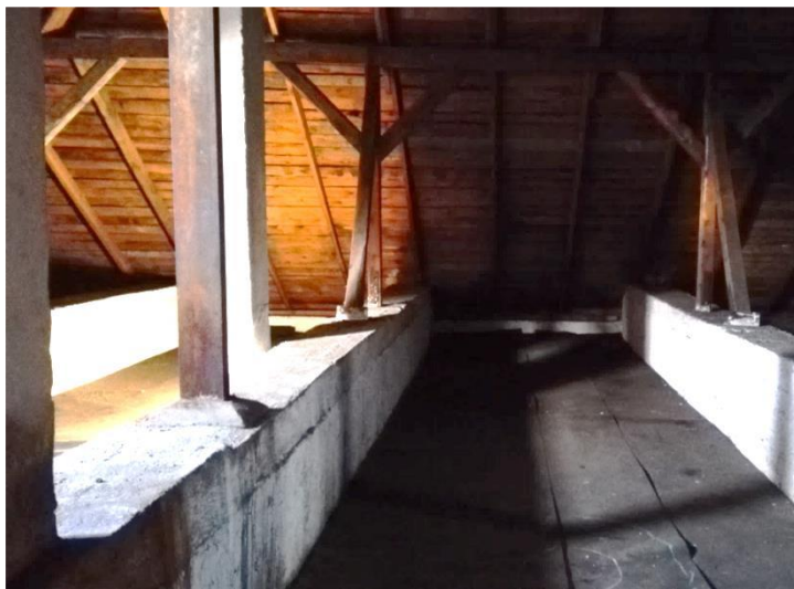
Fig. 20 Example of a reinforced concrete overlay in the ceiling to the unheated loft
