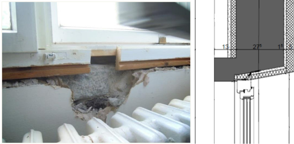
Fig. 19 Hygrothermally critical window connections; left: continuous natural stone window sill from the outside to the inside, right: low wall thickness with additional cross-sectional weakening in the lintel plane.
