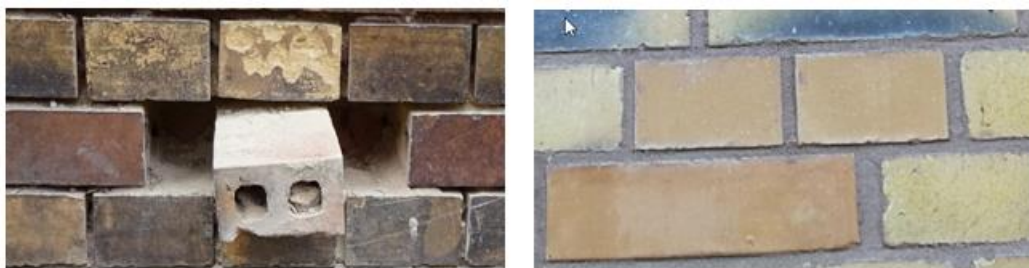
Fig. 8 Existing horizontally perforated brick in the façade: left photo during the as-built analysis, right photo after renovation
