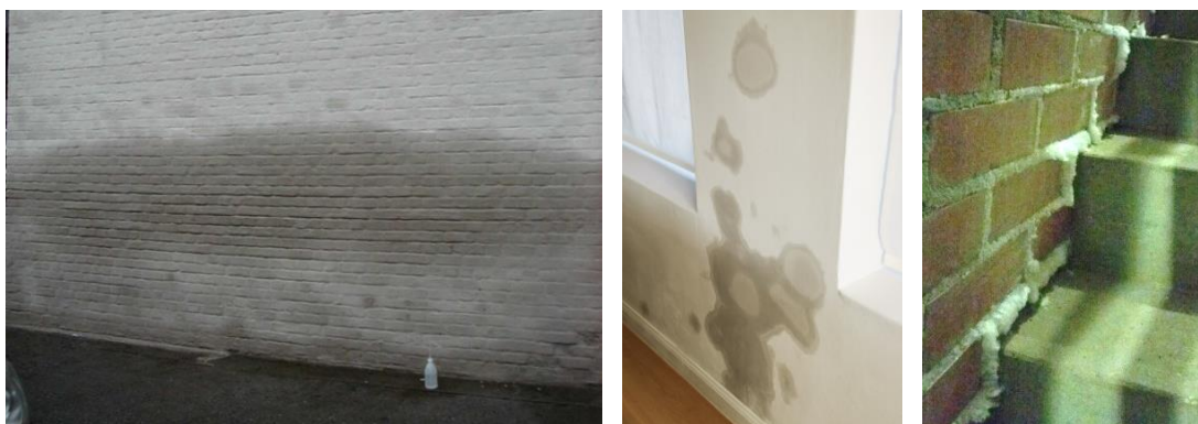
Fig. 12 Hygroscopic moisture and salts on an outer (left) and inner wall (centre); right: on the surface, salt crystallises out
