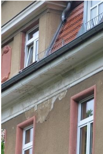
Discoloration on a facade under a rain gutter
