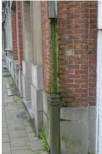
Algae and washed-out mortar due to missing rainwater pipe
