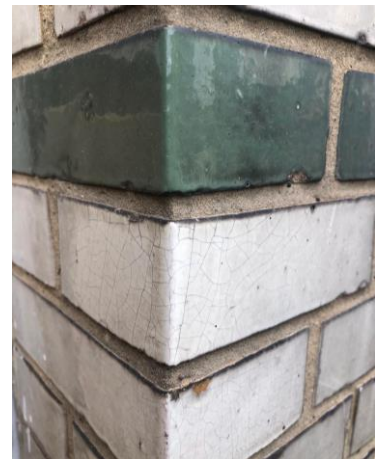
Glazed bricks (early 20th century); masonry can still dry out through the joints in between the bricks
