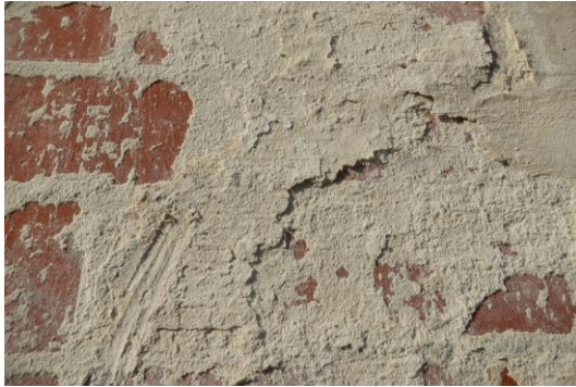
Degradation of a mineral paint
