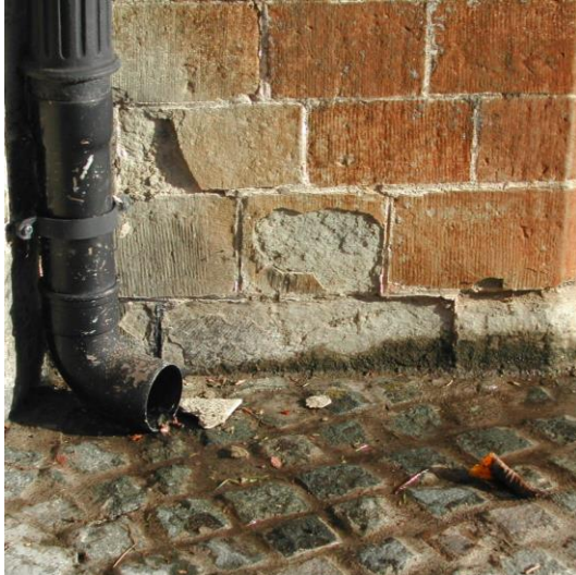
Degradation of natural stone at a wall base, due to wetting and frost.
