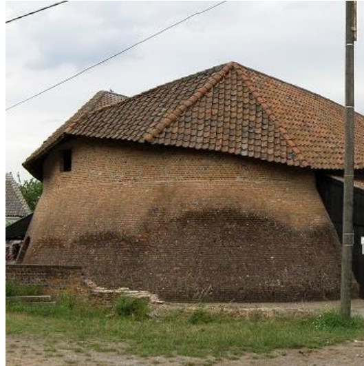
Discolouration of a non-vertical façade due to bacterial growth, caused by rainwater running off a roof without gutter. The bacteria are not the main problem, but a symptom of high rainwater exposure
