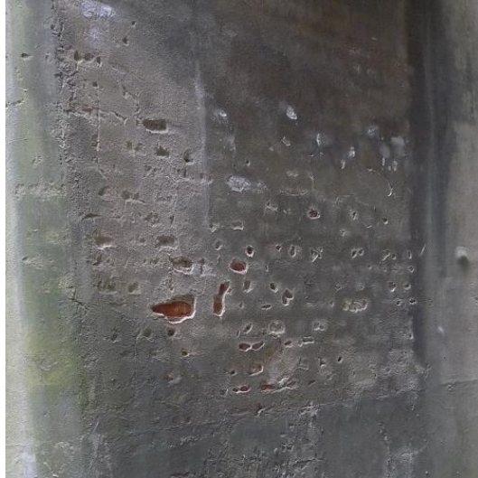
Damage to an exterior render, mainly due to salt crystallisation. The differences in porosity and pore size distribution between render, mortar and bricks give this specific damage pattern.
