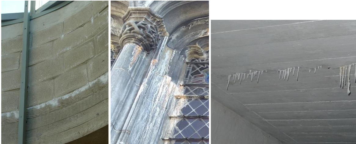
Fig. 9 Often, rainwater infiltration causes \text{Ca(OH)}_2 to be washed out of concrete or mortars and deposited on surfaces where it turns into calcite. Such white run-off, sometimes even visible as stalactites, is a very clear sign of infiltrations. The presence of such run-off indicates a serious problem. It can lead (in concrete structures for instance) up to significant material damage and stability problems (degradation of mortars, increased corrosion of steel reinforcement bars in concrete)
