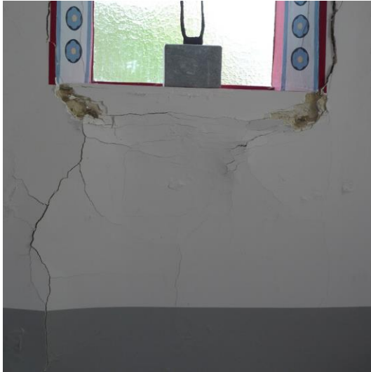
Degradation of plaster due to infiltrations through the façade
