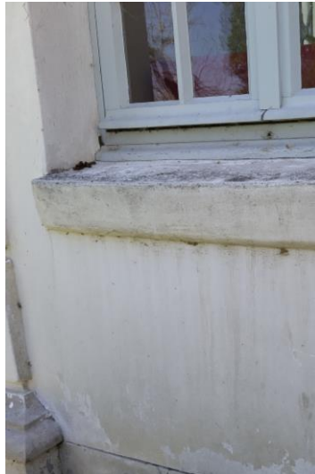
Water run-off on underlying wall demonstrate less efficient protection of non-ideal sill
