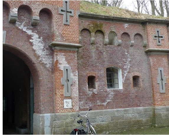
Salt efflorescence due to the drying out of a wall
