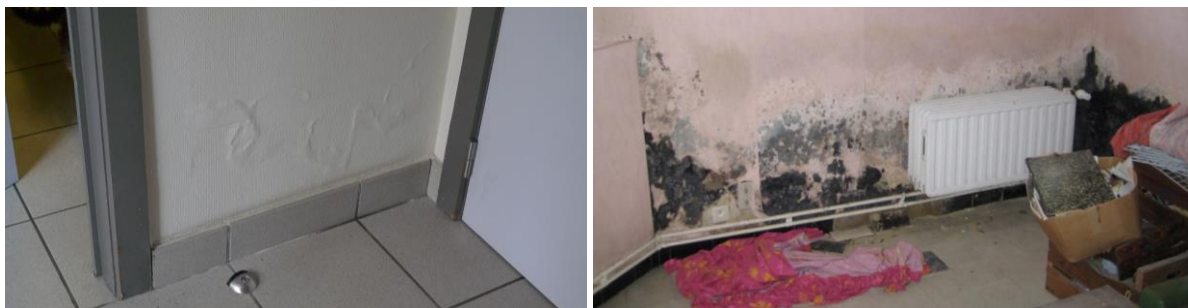
Fig. 10 Rising damp visible on the interior surface of an inner wall (left) and an outer wall (right)
