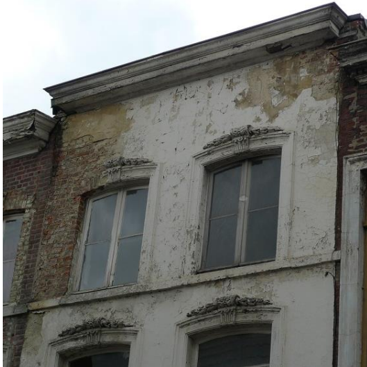
Damage, due to frost, of external render, following the abnormal wetting of the plaster because of a blocked gutter.
