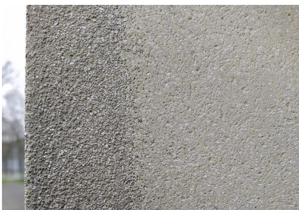
Fig. 8 Different condition of the surface, in this case the washing out of the binder, may indicate differences in driving rain load exposure
