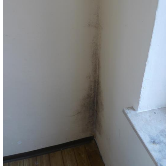
Mould due to low surface temperature in corner of a non-insulated wall
