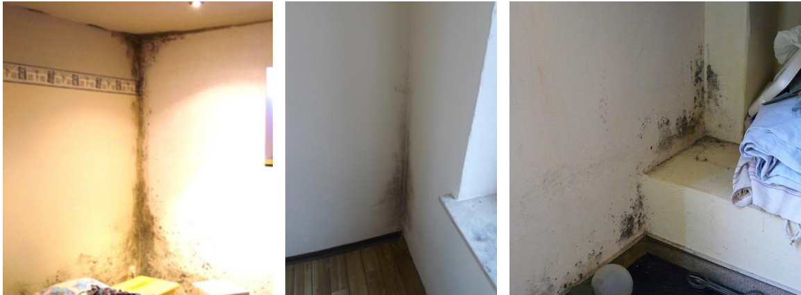
Fig. 13 Mould/condensation in the area of thermal bridges
