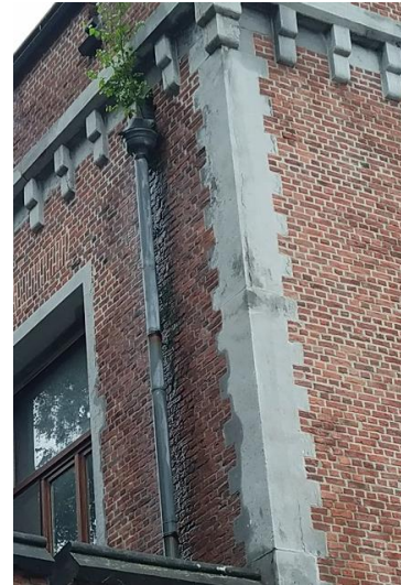
Water running over the façade due to a blockage
