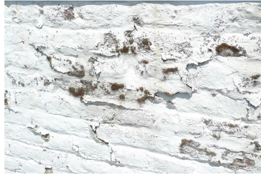
Degradation of a vapour-tight paint
