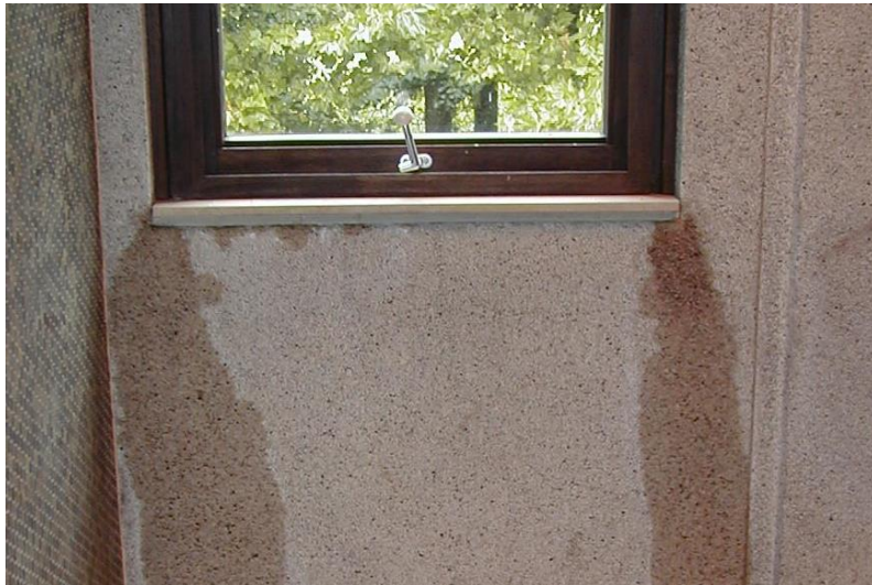
Infiltrations through leaking joints between window and wall
