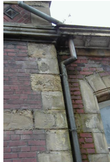
Algae and moss growth due to a defect external downpipe
