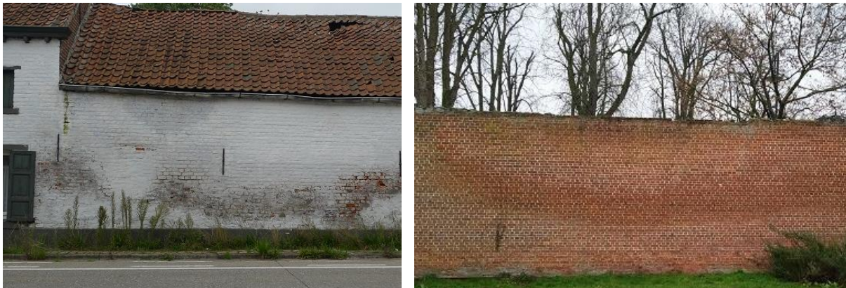
Fig. 11 Purely visually, it is not always easy to distinguish the moisture source. Left: dampening caused by rising damp. Right: dampening caused by hygroscopic salts
