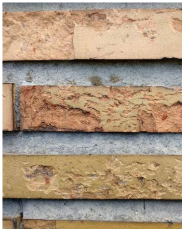
Flaking off of the glazed surface (~1930s)
