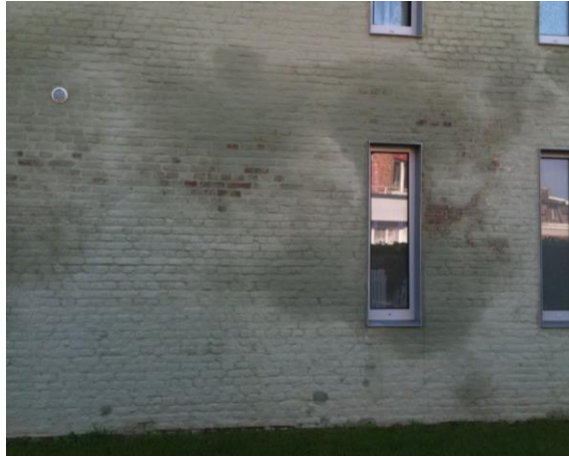
Hygroscopic moisture due to hygroscopic salts
