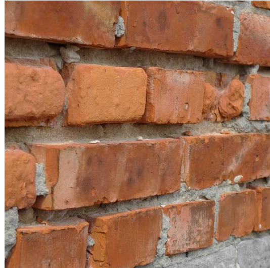
Damaged mortar joints
