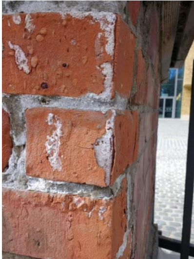
Loss of surface layer because of the application of a water repellent agent on a damp and salt-loaden wall
