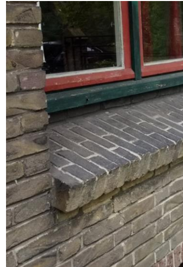
Brick window sills protect underlying wall less efficiently
