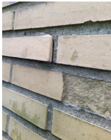
Glazed bricks (~1960s) degrading due to frost and limited drying potential of the masonry
