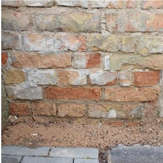
From the surface, the bricks crumbles away
