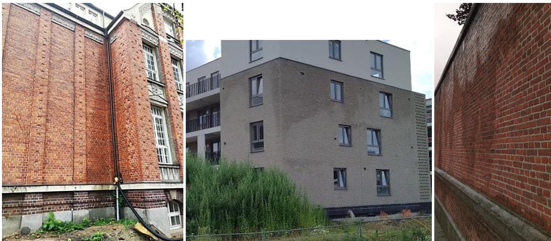
Fig. 5 Inspection after a rain event to visually check the moisture distribution on façade surfaces. Left: visible moisture load due to defective temporary rain water downpipe; middle/right: exposed parts become visible
