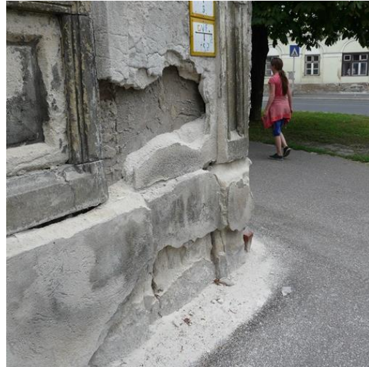
No adhesion between plaster and base. The plaster crumbles away
