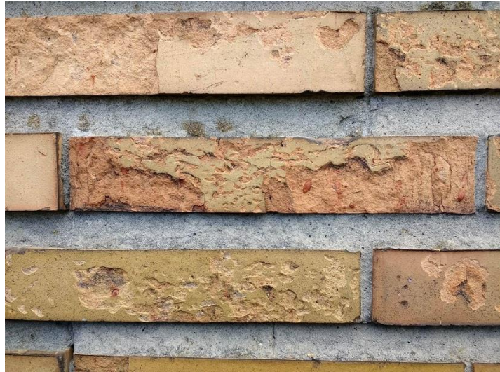
Loss of salt glaze because of frost of the damp material behind the dense finishing layer
