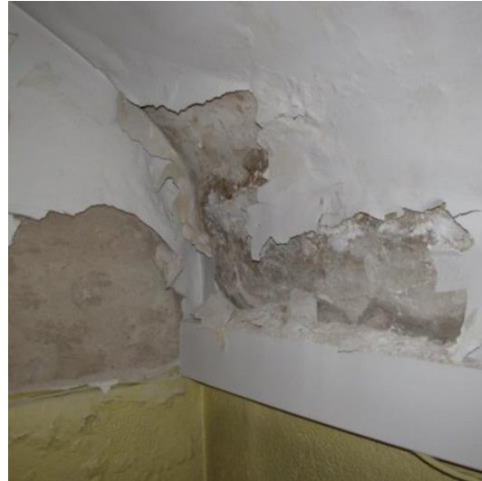
Coating and plaster are spalling off
