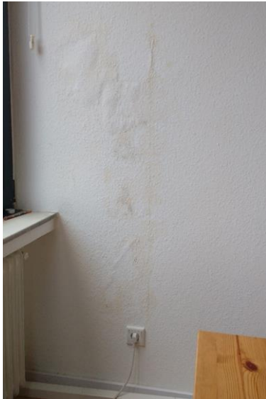
Damp spot in room, partly detached wallpaper
