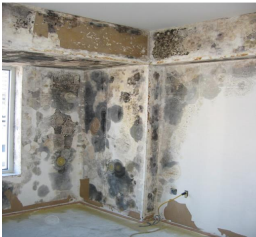
Fig. 14 Significant mould growth behind a removed PVC wallpaper (Wiss J. Elstner Associates, Inc.)
