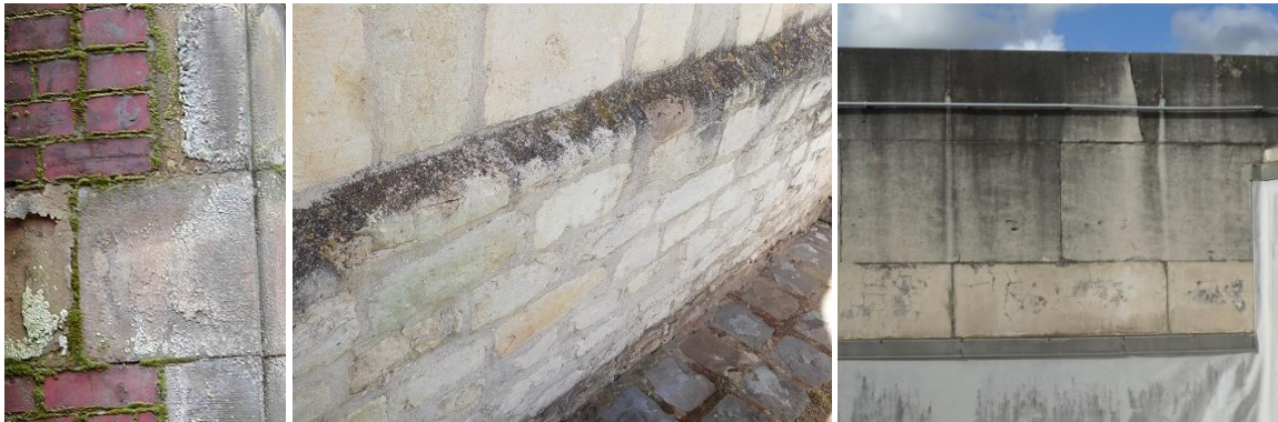
Fig. 6 Biological growth of moss, algae and bacteria showing where facades are exposed to rainwater
