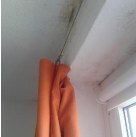
Mould due to thermal bridges (window opening and ceiling connection)
