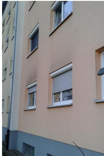
Bacteria growth above window lintels
