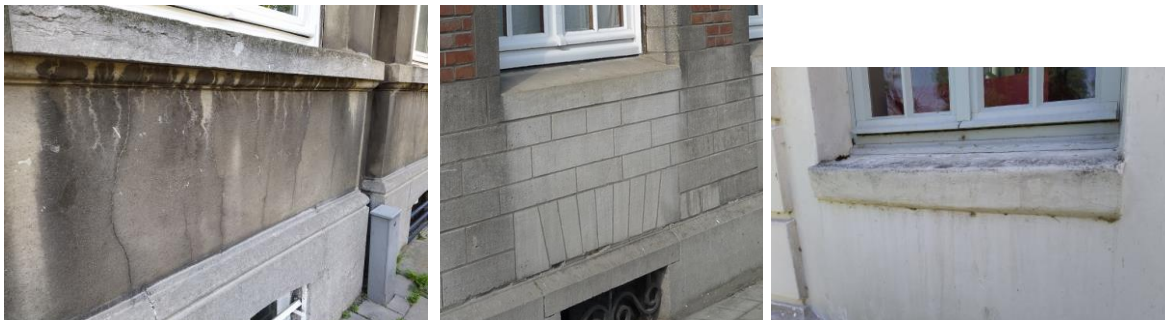
Fig. 7 Differences in pollution under a window sill. Left: apart from some runoffs, the surface under the window sill is well protected from water, as it is sooty; middle: cleaner surface under the sill, indicating it is exposed to rain; right: the runoffs of water under the sill can easily be observed
