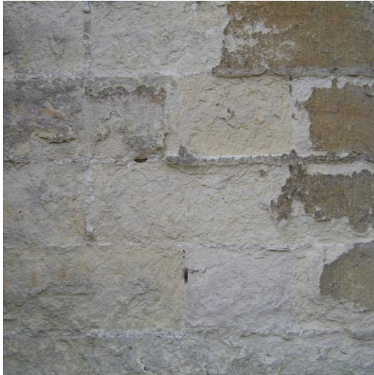
Degraded limestone due to acid rain
