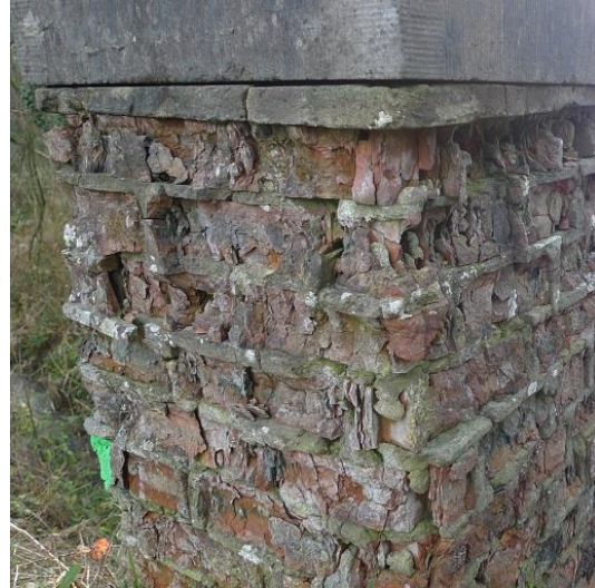
Degradation of bricks, due to abnormal wetting (the capstone is not designed well) and frost.
