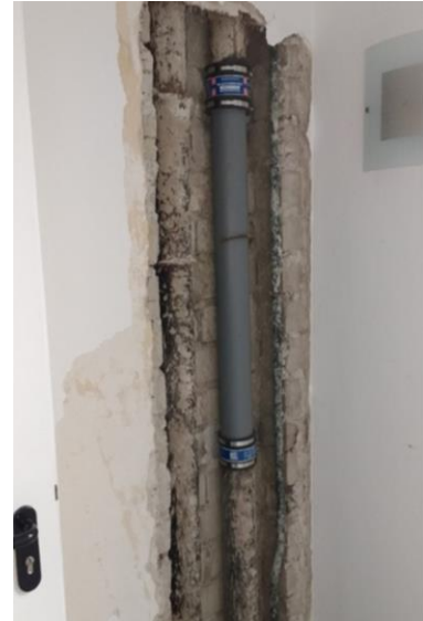
Replaced internal pipe
