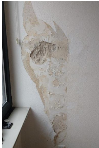
After removing wall paper visible mould stains
