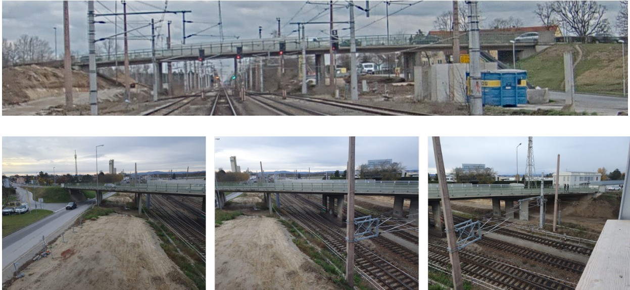
Figure 25: Road bridge in Deutsch-Wagram, L13 Bockfließersstraße over the ÖBB before demolition
