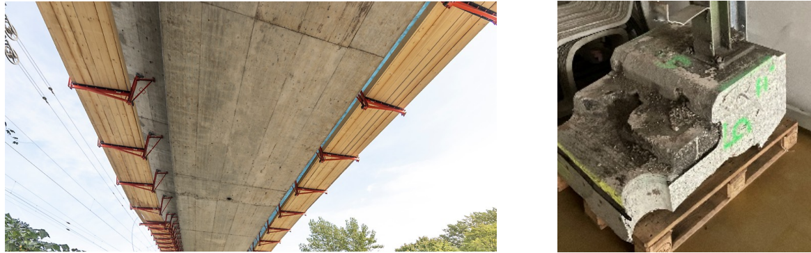
Figure 28: Renovation of the bridge support structures of the Vienna West Exit with demolition of the edge beams and production of a concrete topping (left), edge beam cross-section for sampling in the FHCW laboratory (right)
