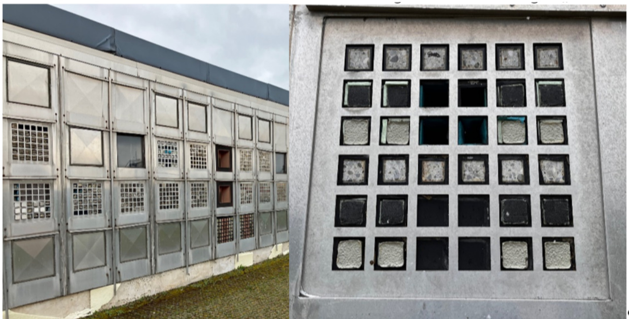
Figure 79: Field test facility in Holzkirchen with west orientation with strong driving rain load Left: CRUFI specimens are exposed at 2m height. Right: detailed built in situation.
