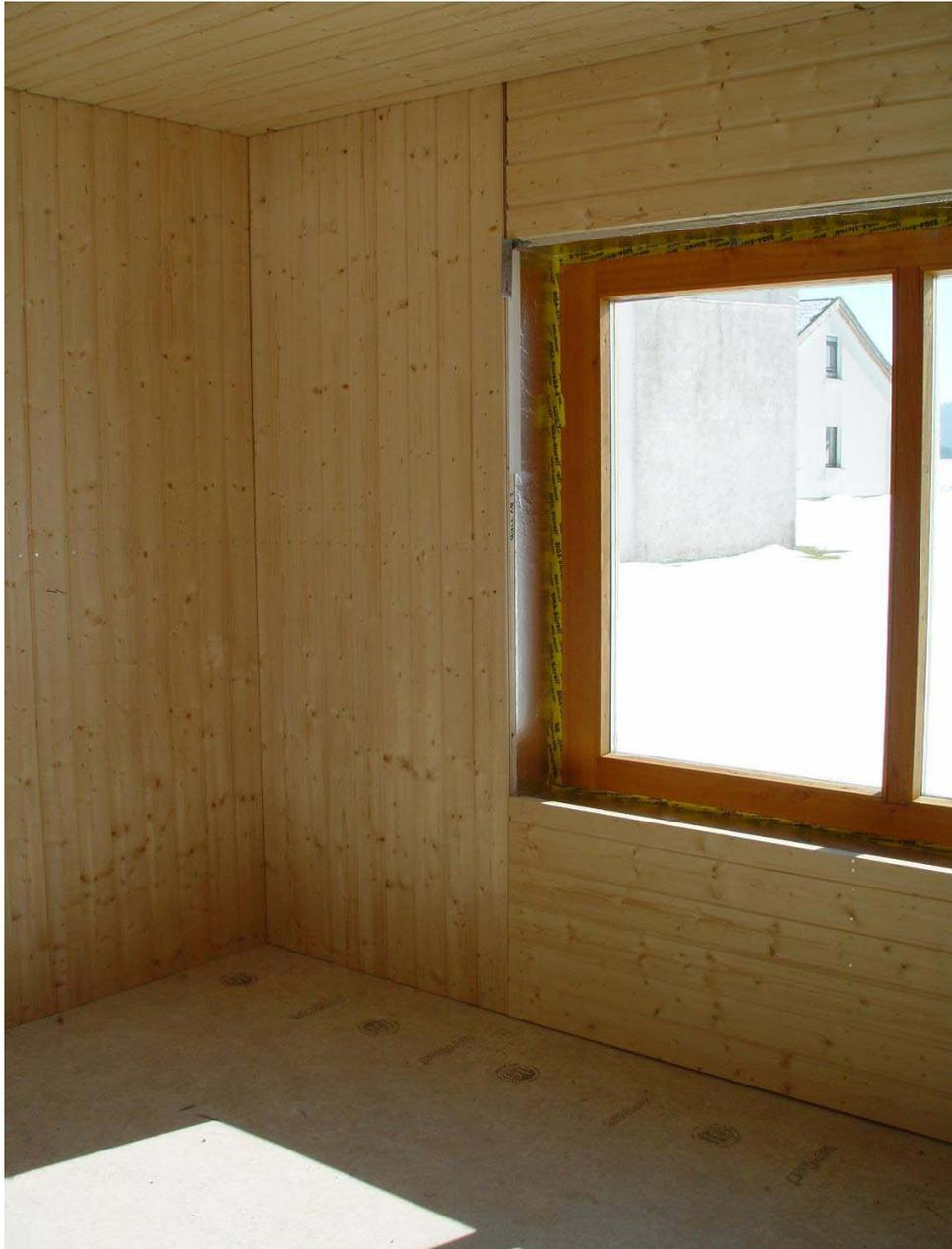
Fig. 25: Test room with spruce panels.
