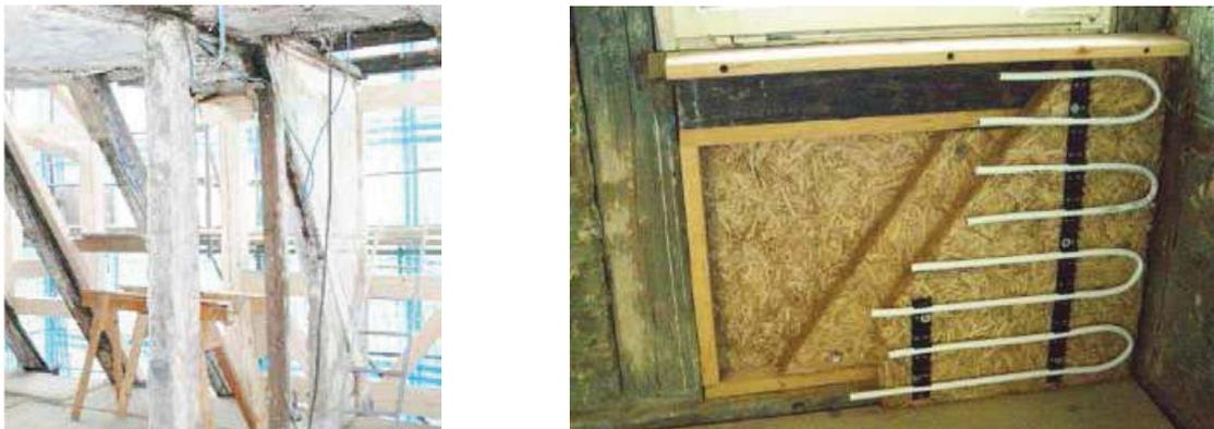
Fig. 2. Condition of the wooden framework before restoration (left) and scheme of the insulation (right), pictures by Alexandra Fritsch.
