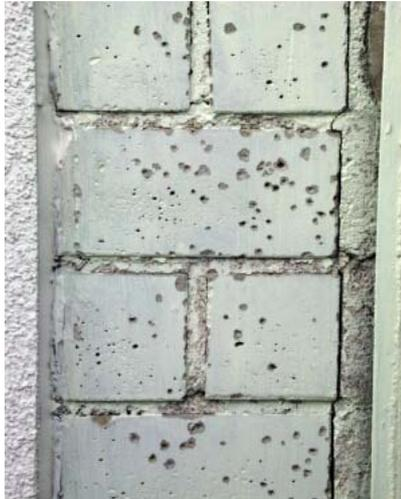
**FIGURE 1:** Photograph of frost damage on a west-facing calcium silica brick wall at the outdoor testing field at the Holzkirchen IBP site following the 1998/99 winter.
